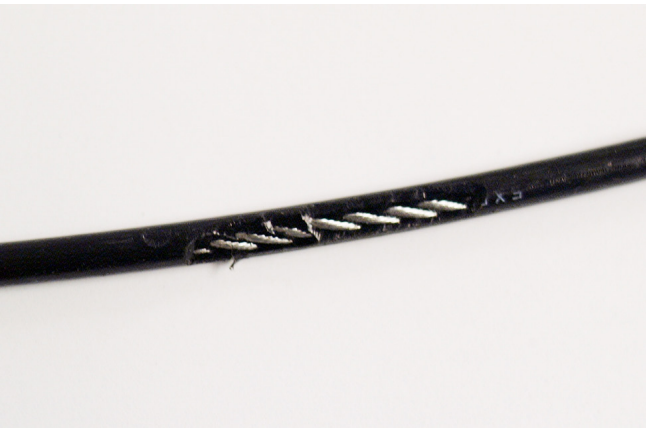
A TEAR IN THE CABLE COVER
